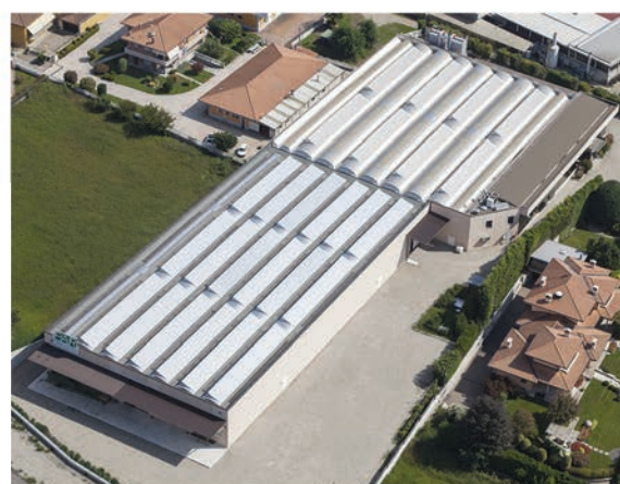
FAR - New factory in Gozzano (NO)
